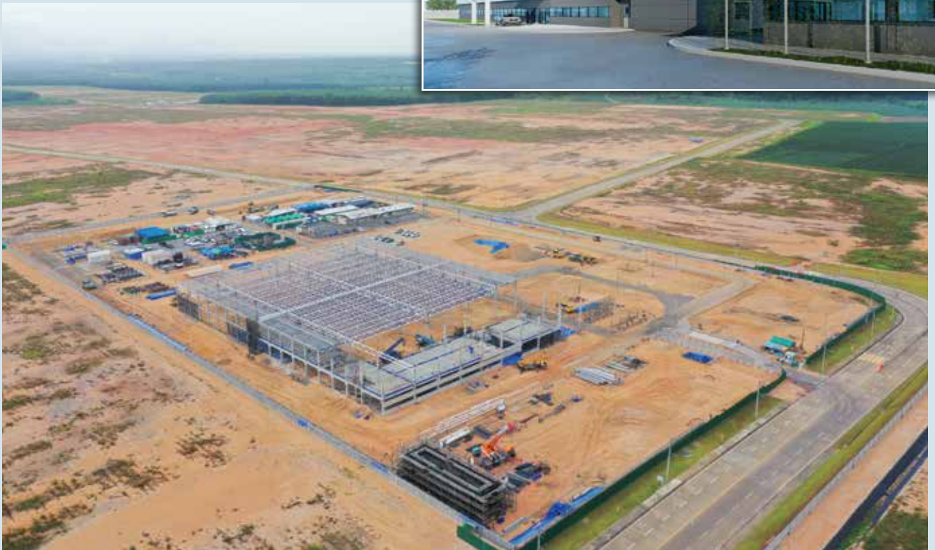
Top: A rendering of CoorsTek's finished plant in Thailand. Bottom: Construction proceeds on CoorsTek's Thailand plant. Credit: CoorsTek Inc.
