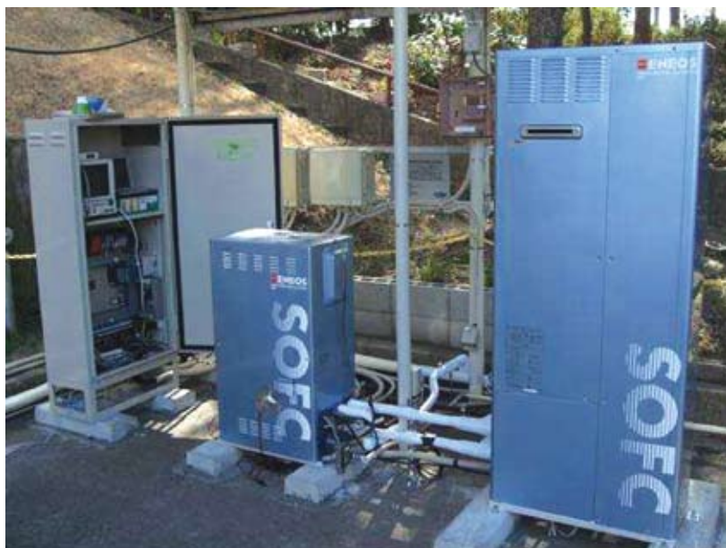
Fig. 1. SOFC-based residential combined heat and power system showing the SOFC unit (left) and the hot water tank (right).
