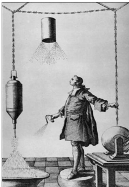
**Fig. 1: Electro spraying devices used for entertainment purposes. Published in *Essai Sur L' El électricité Des Corps* in 1746.**
