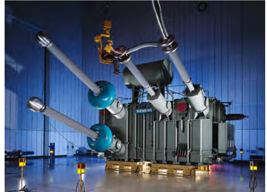
Transformer for High-voltage direct current transmission (HVDC)
