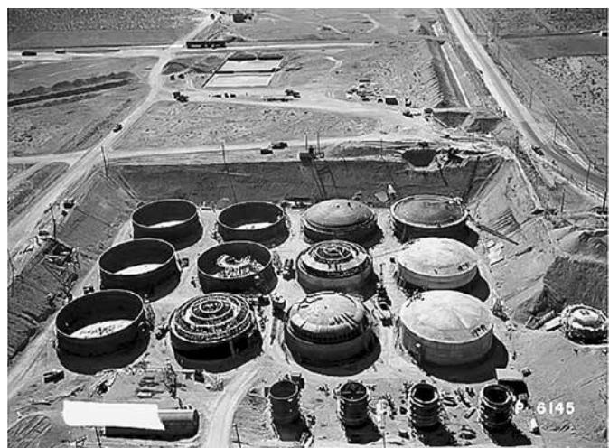
Figure 1. 1943 construction of nuclear waste tanks at the Hanford site. These tanks were designed with a 20-year lifetime, although some waste (including the waste stored in the above tanks) was later relocated to tanks with a 50-year lifetime. 1
