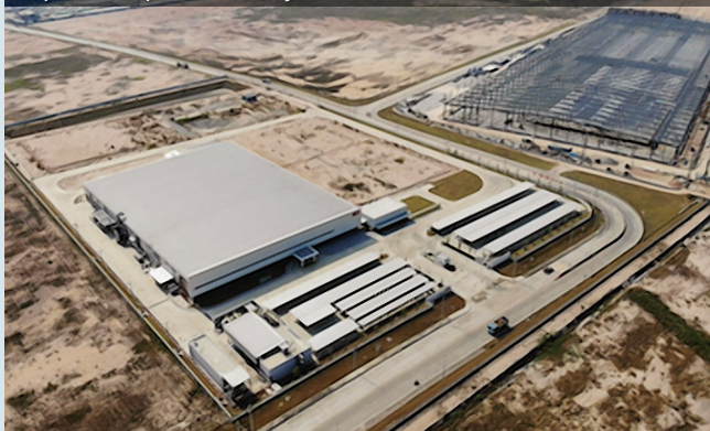
The CoorsTek facility in Rayong, Thailand, where a rooftop and carport solar photovoltaic system will be installed. Credit: CoorsTek
