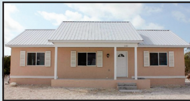
Figure 3. The first Neuskyns nanoceramic housing designed for hurricane resilience in the Caribbean. Credit: NanoArchitech.
