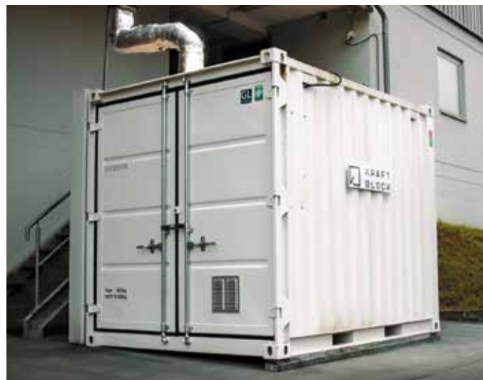
Figure 4. Example of a 10-foot Kraftblock storage that can store 4.2 MWh of waste heat at a max 600°C.
