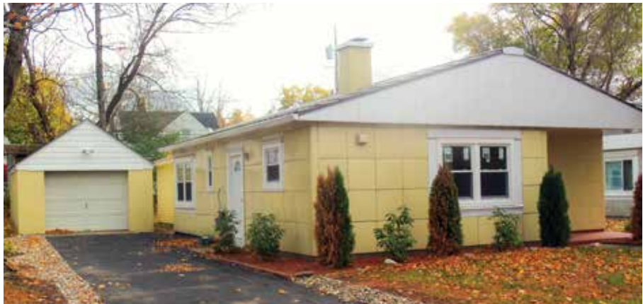
Figure 8. A porcelain enamel Lustron house still stands in Albany, N.Y. From 1948–1950, the Lustron Corporation used an assembly line in a former warplane manufacturing factory in Columbus, Ohio, to manufacture porcelain enamel houses as a quick and low-cost solution to the post-World War II housing crisis.
