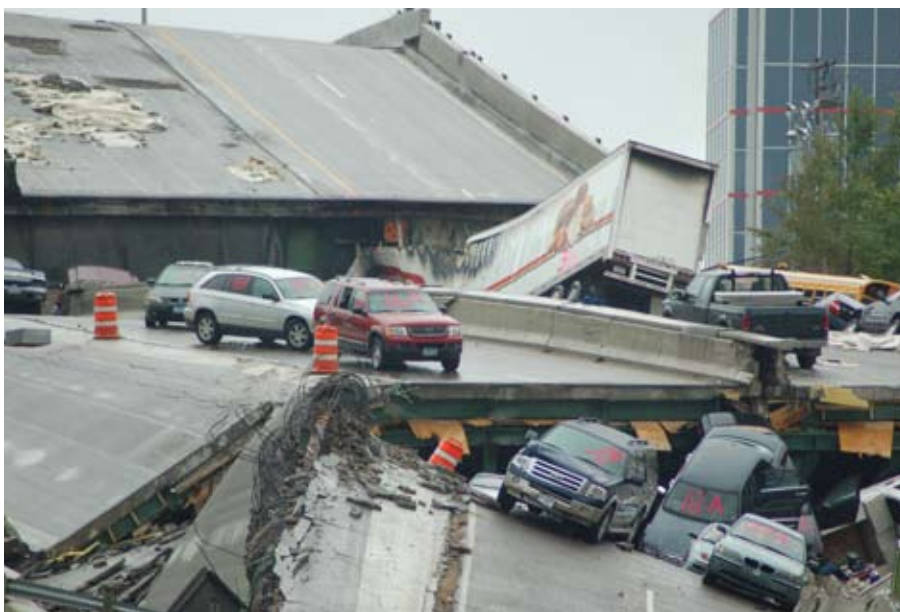
Embedded sensor systems, powered by energy-harvesting materials, can monitor bridge stresses such as those that led to the 2007 bridge collapse in Minneapolis, Minn., and trigger warnings before they occur.
