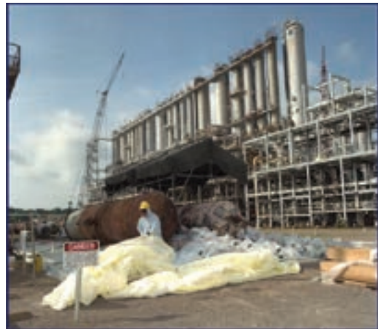
Figure 4. Typical disposal of Asbestos covered steam pipes.
